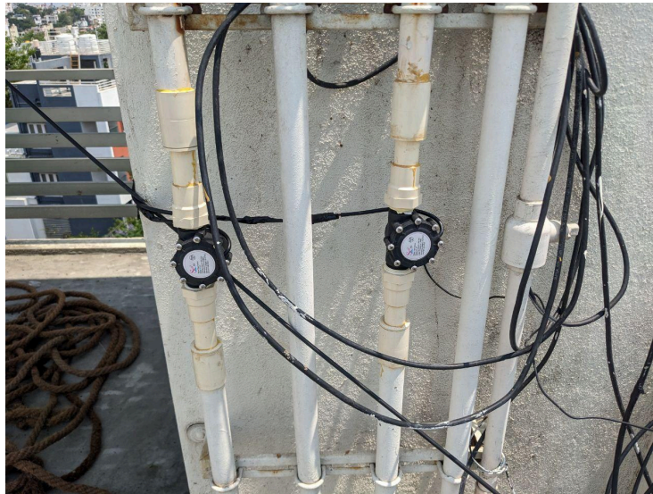
Flow Sensor Installed in House
